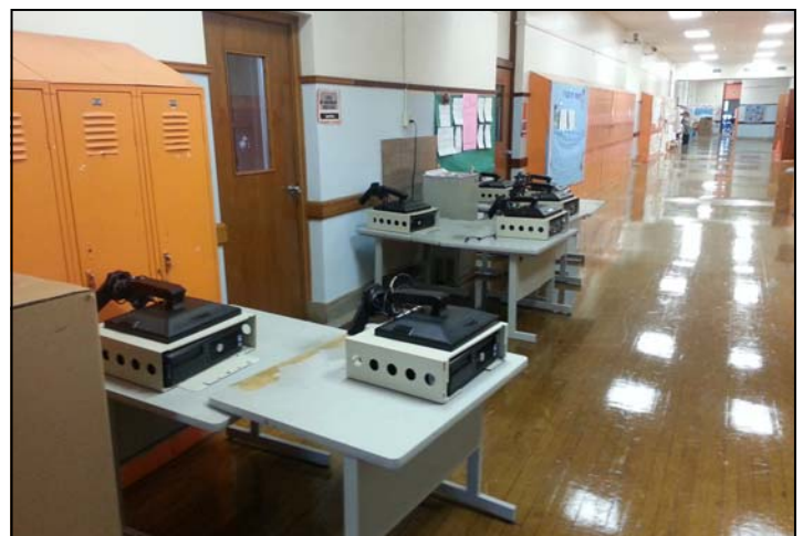
Installation of Dell Optiplex 790's in room 210, freed 25 Optiplex 780's with flat-screen monitors and furniture to the library, a tutoring center, and classrooms throughout the building. The machines were only a year old and in like-new condition.
